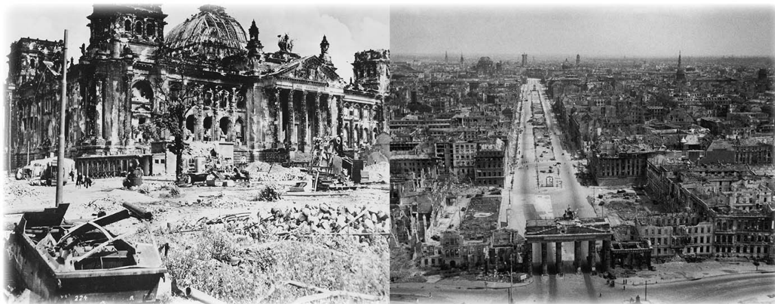
Figure 13.2: Destruction in Berlin: The Reichstag building (left) and the Brandenburg Gate (right).
