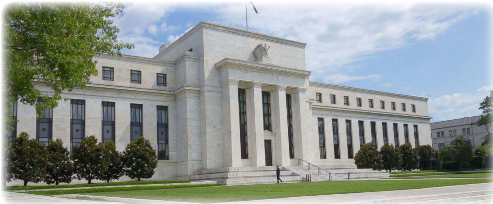
Figure 5.20: The third Bank of the United States, the Federal Reserve. Shown is just one of the 12 Banks part of the system.
