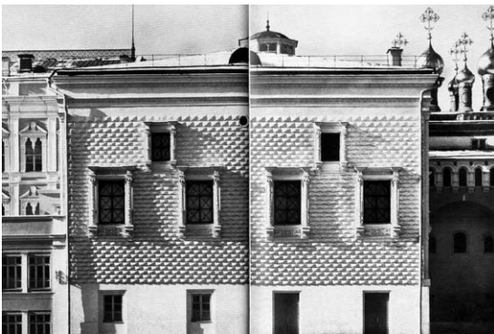
Fig. 3.33. The Faceted Chamber of Kremlin in Moscow. We see the eastern front part of the chamber’s outer wall with faceted blocks of stone, hence the name. Taken from [191], inset.
