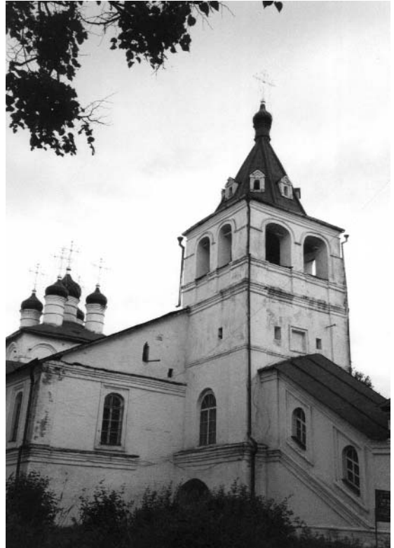
Fig. 14.157. The Ouspenskaya Church at Alexandrovskaya Sloboda (the modern town of Alexandrov). See also [11].
