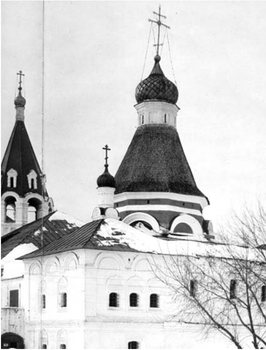
Fig. 14.152. The dome of the Pokrovskaya Church. Taken from [1373], pages 68-69.
