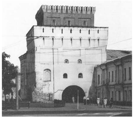
Fig. 14.2. The Vlassyevskaya, or Znamenskaya tower that had formerly been part of Yaroslavl’s sturdy fortifications, destroyed in the Novgorod pogrom (according to our reconstruction). A view from the west. Modern photograph. Reproduced in accordance with [996], page 73. In the left corner of the Znamenskaya Tower one can clearly see the remnants of a brick wall, which had once stood adjacent to the tower. The wall was destroyed – there is nothing left but uneven marks.
