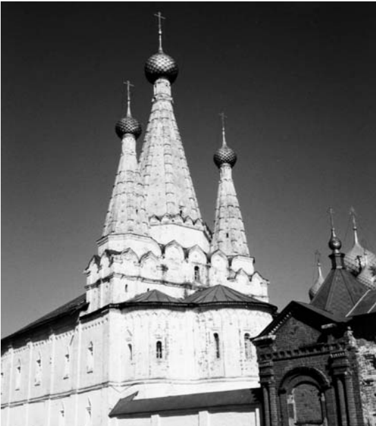
Fig. 14.222. Church of Metropolitan Alexei in Ouglich. View from the southeast. Photograph taken in 2000.
