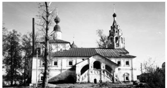
Fig. 14.224. The Church of Presentation, the Nikolo-Ouleimskiy Monastery, Ouglich. Northern view. The church is entered via a tall porch that leads directly to the first floor. Photograph taken in 2000.
