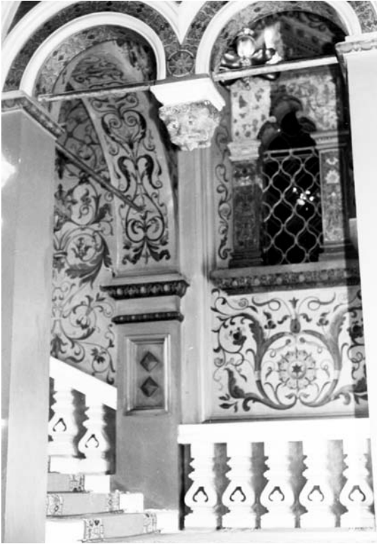
Fig. 14.203. Staircase to the fourth floor of the royal harem (Teremnyy Palace) of the Muscovite Kremlin. Photograph taken by the authors in 2000.
